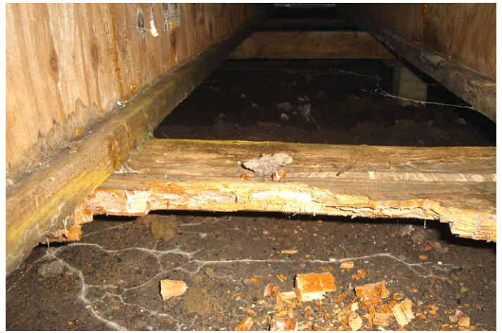
VIEW BETWEEN I-BEAM JOISTS: STYRENE/FOIL REMOVED
