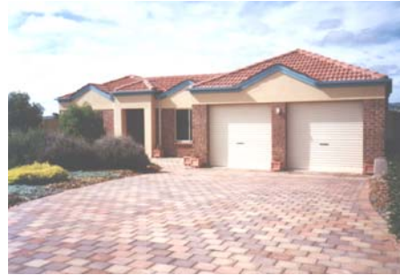
Figure 2: A standard project home
