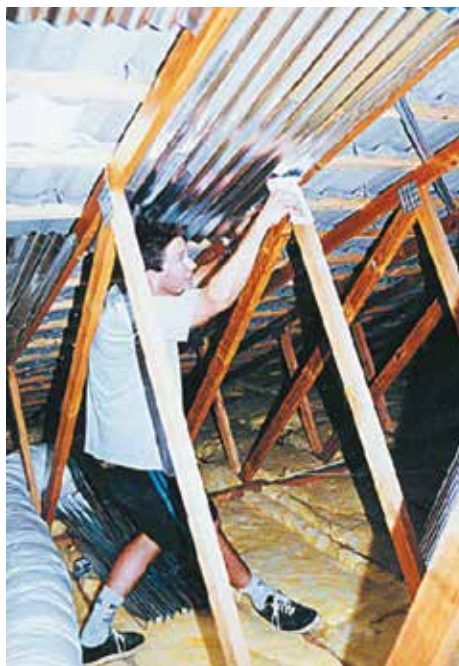
Concertina FOIL BATTs stapled between rafters protects air-conditioning ductwork from intense heat radiating from the roof
